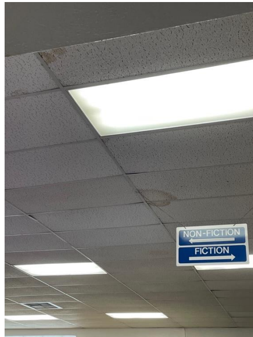
Figure 1 – Water-Stained Ceiling Tiles
