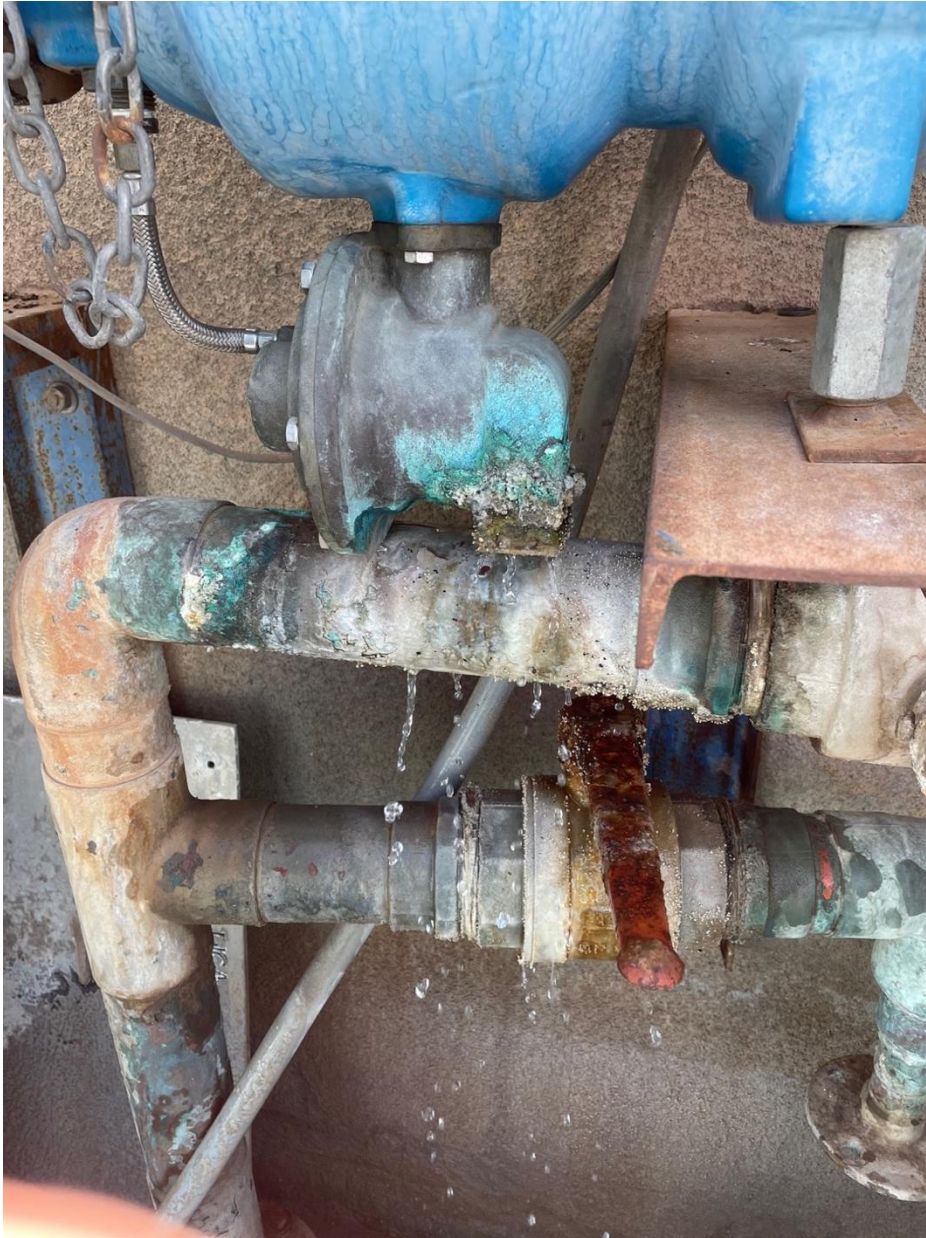
Figure 4 – Leaking Backflow Prevention Device
